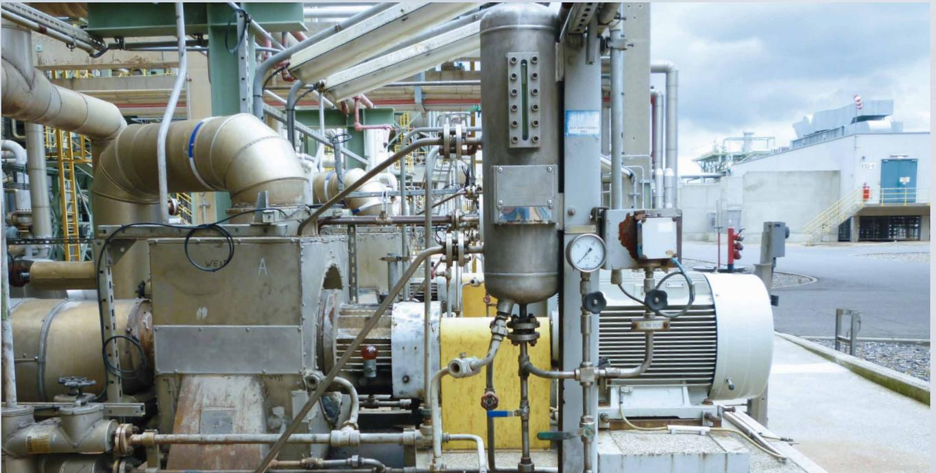
IDP pump with seal supply unit in application at TOTAL Leuna.
