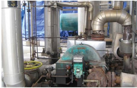
Boiler feed water pumps in the hydrogen unit of the Turkish Tüpras Kirikkale refinery are equipped with EagleBurgmann **SHPV2/64** seals and supply systems to API 682 Plan 02 + 23. Operating conditions:  $p = 43 \text{ bar}$  (624 PSI);  $t = \dots 282 \text{ }^\circ\text{C}$  (540 °F);  $n = 1,470 \text{ min}^{-1}$ ;  $d1 = 58 \text{ mm}$  (2.28"). Medium: boiler feed water
