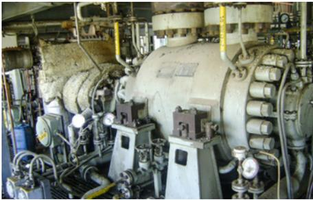
A high pressure dry gas seal EagleBurgmann type **PDGS2.1/130** seals a Bhel compressor in the hydrocracker unit of the Panipat refinery in India. Operating conditions:  $p = \dots 179 \text{ bar (2596 PSI)}$ ;  $t = 160 \text{ }^\circ\text{C (320 }^\circ\text{F)}$ ;  $d_1 = 112 \text{ mm (4.41")}$ . Media: H<sub>2</sub> + CH<sub>4</sub>, N<sub>2</sub>.
