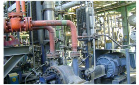
For a KSB pump installed in the delayed coker unit, the Indian Panipat refinery applied EagleBurgmann pusher seals **LL9DTUU** in tandem arrangement. Operating conditions:  $p = 23.5 \text{ bar (340 PSI)}$ ;  $t = 40 \text{ }^\circ\text{C (104 }^\circ\text{F)}$ ;  $n = 2,900 \text{ min}^{-1}$ ;  $d1 = 58 \text{ mm (2.28")}$ . Media: hydrocarbons.
