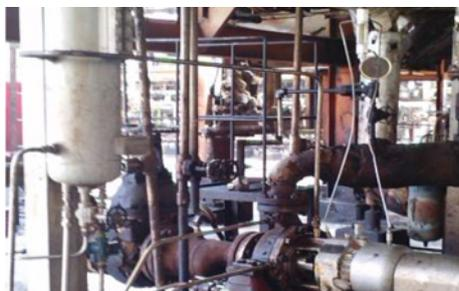
In the distillation unit of a Mexican refinery in Salina Cruz, Oaxaca, EagleBurgmann metal bellows seals type **MFLWT80/75** seal the shafts of Sulzer horizontal pumps. Operating conditions:  $p = \dots 9.42 \text{ bar (137 PSI)}$ ;  $t = 175 \text{ }^\circ\text{C (347 }^\circ\text{F)}$ ;  $n = 3,560 \text{ min}^{-1}$ . Media: hydrocarbons
