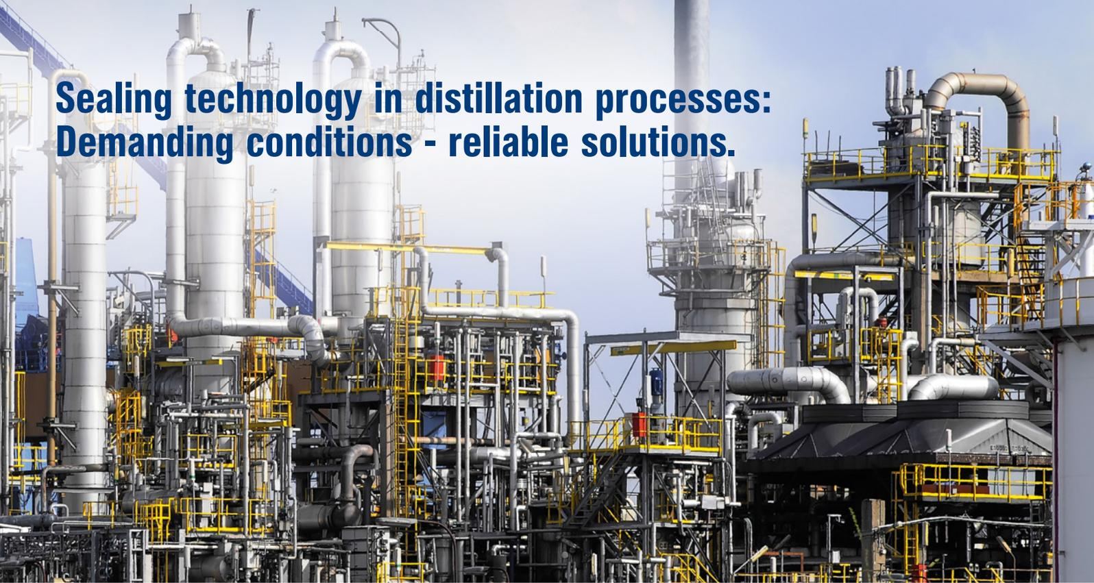
For distillation, the crude oil is first heated to around 350 °C (662 °F) and then broken down into individual products. Substances with a boiling point above this temperature become gaseous and rise in the distillation column.
