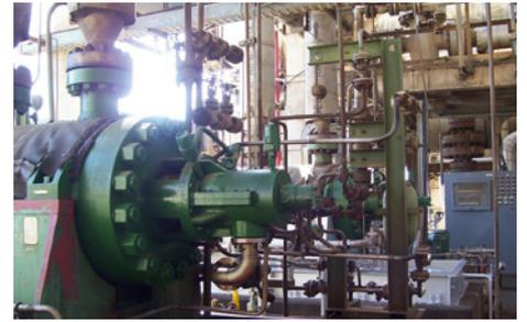
**H75KF-D1/130** back-to-back dual seals with supply system **SP09030/M012-D1** to API 682 Plan 53 have been successfully sealing the shafts of Pacific between bearing pumps since 2004. The system is located in the CRP refinery of Petroleos De Venezuela S.A. Operating conditions:  $p = 4 \text{ barg}$  (58 PSIG);  $t = 200 \text{ }^\circ\text{C}$  (392 °F);  $n = 3,600 \text{ min}^{-1}$ ;  $d1 = 104.1 \text{ mm}$  (4"). Media: naphtha, gasoil + 3 %  $\text{H}_2\text{S}$ .
