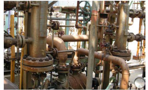
The shafts of KEPL pumps of Chennai Petroleum Corporation Ltd. in India are reliably sealed by EagleBurgmann metal bellows seals type **MFLWT80/90** and **MFL65F/85**. Operating conditions:  $p = 16.08 \dots 19.93 \text{ bar (233 } \dots 289 \text{ PSI)}$ ;  $t = 238 \text{ }^\circ\text{C } \dots 263 \text{ }^\circ\text{C (460 }^\circ\text{F } \dots 505 \text{ }^\circ\text{F)}$ ;  $n = 2,955 \text{ min}^{-1}$ ;  $d_1 = 80 \text{ mm (3.15")}$ . Media: hydrocarbons.
