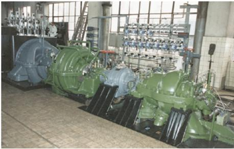
Coking oven gas compressor (Mannesmann Demag) at Wintershall AG, Lingen. Originally equipped with labyrinth seals, the turbine-driven single-shaft radial compressor has been converted to EagleBurgmann dual **DGS** seals and a buffer gas supply system. Operating conditions: p = 5.6 barg (81 PSIG); n = 12,800 min<sup>-1</sup>; d1 = 134.8 mm (5.3"). Medium: gas with H<sub>2</sub>S content.
