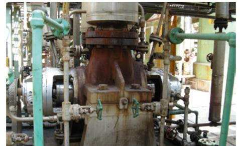
EagleBurgmann **LL9DTUU** dual mechanical seals are applied to seal a Sulzer pump of a catalytic cracking unit operated by Chennai Petroleum Corporation Ltd. in India. Operating conditions:  $p = \dots 13.73 \text{ bar (199 PSI)}$ ;  $t = 40 \text{ }^\circ\text{C (104 }^\circ\text{F)}$ ;  $n = 2,965 \text{ min}^{-1}$ ;  $d_1 = 70 \text{ mm (2.7")}$ . Media: hydrocarbons.
