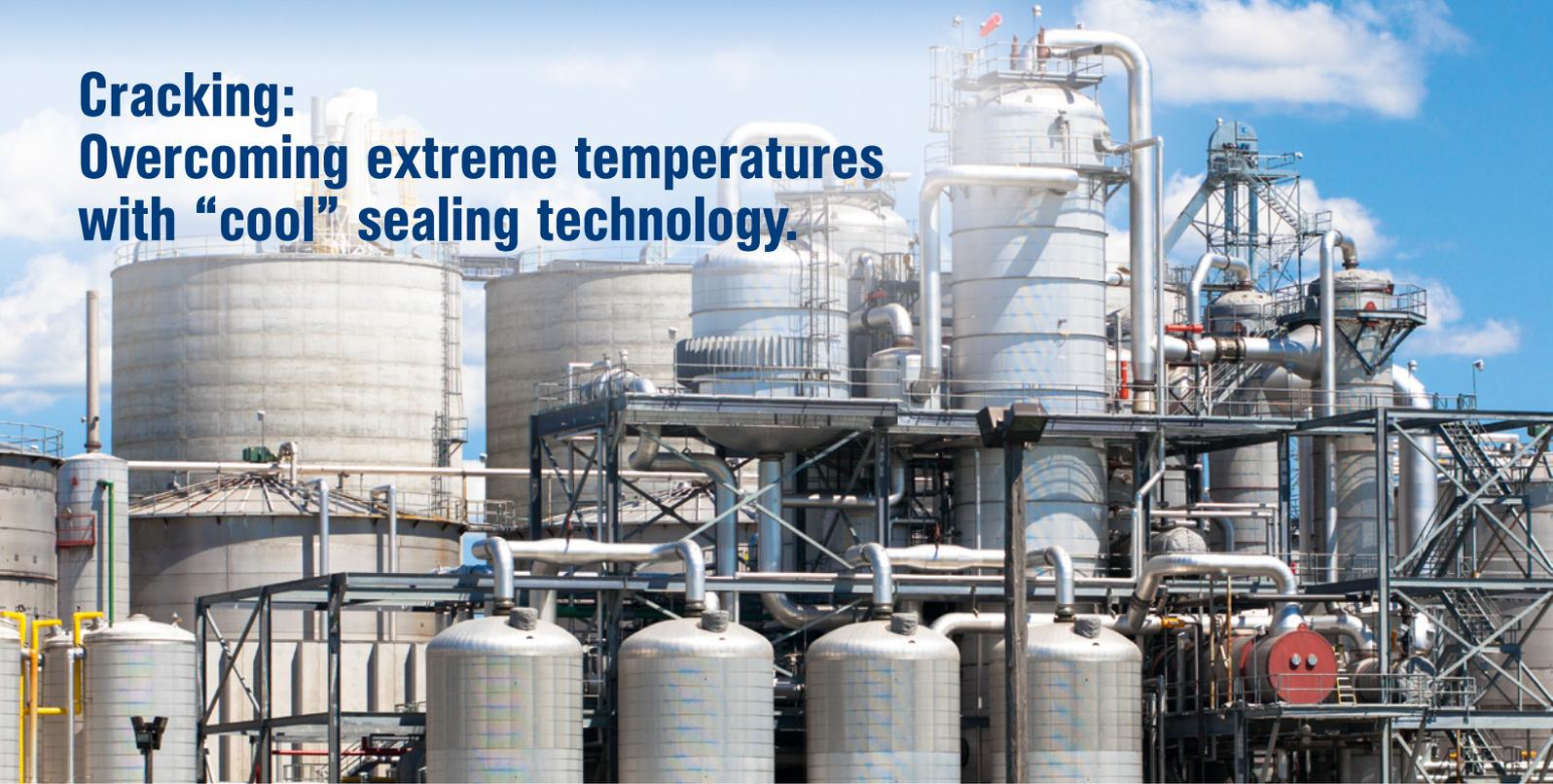
The fraction of crude oil which cannot be distilled further is then cracked. In this process, long chain molecules are split into smaller molecules under pressure and temperature in order to generate additional short-chain hydrocarbons such as gasoline, diesel or kerosene.
