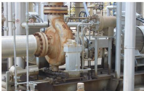
**MFLWT80F2/85** mechanical seals with a **WEL** air fin cooler to API 682 Plan 21, installed in a bottom pump-around pump from Sulzer in the distillation unit of the Sohar refinery in Oman. Operating conditions:  $p = \dots 4.19 \text{ barg (60 PSIG)}$ ;  $t = 278 \text{ }^\circ\text{C (532 }^\circ\text{F)}$ ;  $n = 1,475 \text{ min}^{-1}$ ;  $d_1 = 68 \text{ mm (2.68")}$ . Medium: gas oil.
