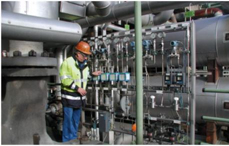
For a MAN Turbo compressor at Shell Godorf, Germany, EagleBurgmann has supplied a **DGS20/113** dry gas seal together with a **SMS** seal management system. The compressor is operated in the gas processing section of the plant. Operating conditions: p = ... 30 bar (435 PSI); t = -20 °C ... 180 °C (-4 °F ... 356 °F); n = 9,811 min<sup>-1</sup>; d1 = 100 mm (3.94"). Medium: gas.
