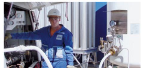
Sealing of tank loading and unloading pumps with **MFLS12** metal bellows seal. The low temperatures demand the application of special seal face and secondary sealing materials with BAM approval. Typical operating conditions:  $p = 5 \text{ bar}$  (73 PSI);  $t = -190 \text{ °C}$  (-310 °F);  $n = 6,000 \dots 8,000 \text{ min}^{-1}$ .
