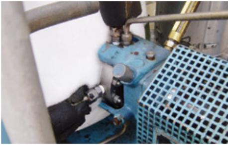
Liquid, high-purity ethylene is pumped in the cracker operated by the Dow Olefinverbund in Böhlen, Germany. The pump shaft is sealed by a **MFLCT80S1** type triple seal. The metal bellows seal has clear benefits at the temperatures down to  $-100\text{ °C}$  ( $-148\text{ °F}$ ) encountered in this environment. A **TS2000** type Thermosiphon system supplies the seal.
